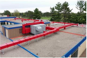
outside air being brought into a building based on the temperature and relative humidity of the air both indoors and out. Outdoor air units are also used to bring in more outside air. They have been developed to produce a lower airflow rate than average. Considering it is solely outdoors, an ancillary HVAC system should also be present to still control the indoor space's temperature and humidity. The most common ancillary system is Demand Controlled Ventilation (DCV),
